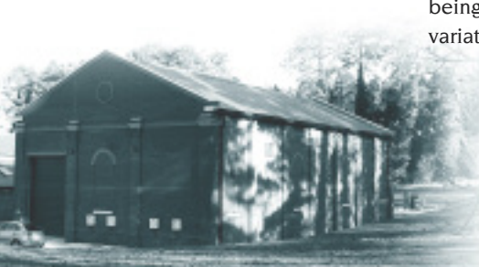
Soberton filtration building
