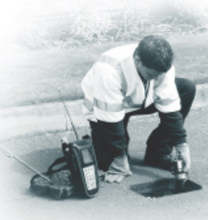
Inspector installing leak location sensors
