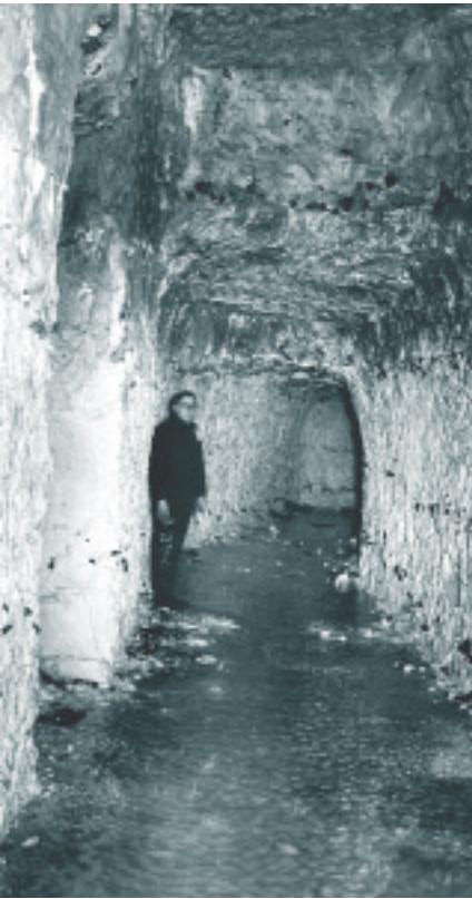
Groundwater in chalk adits at Maindell source, Fareham, 1954
