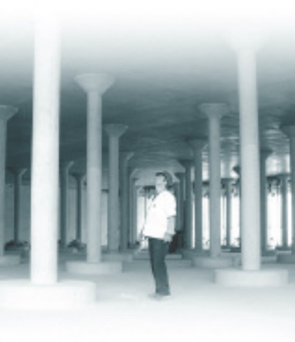
During construction of Farlington No.8 service reservoir
