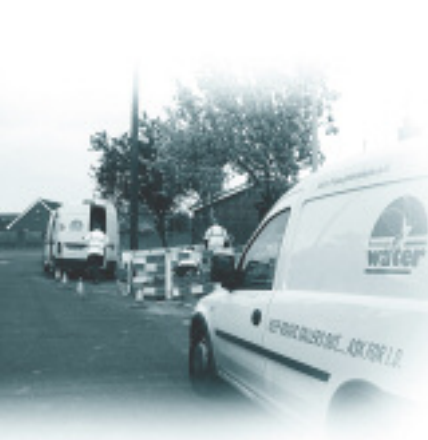
A burst main being repaired
