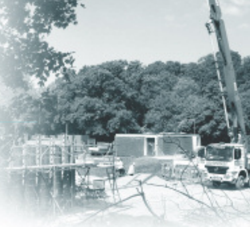
Construction of Westergate Borehole head works
