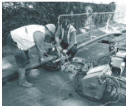
Butt fusion welding equipment for jointing polyethylene pipes
