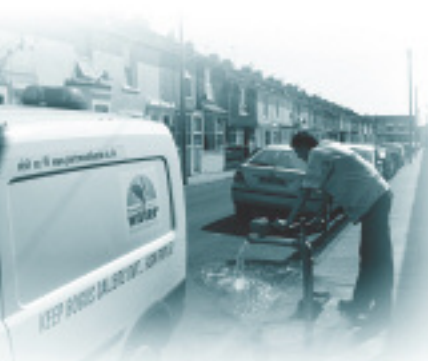
Mains flushing in Copythorn Rd, Portsmouth
