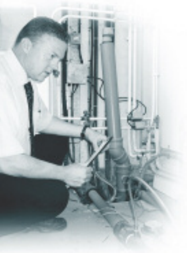
Inspecting plumbing for water regulation compliance
