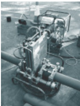
Butt fusion welding in progress
