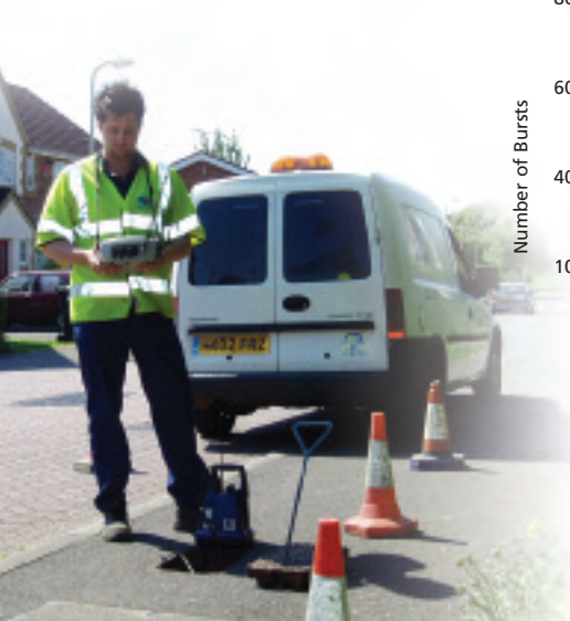
Installing leak location sensors
