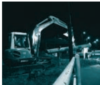
Main laying at Hayling Island bridge
