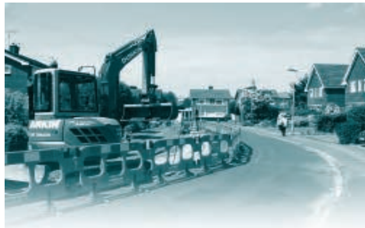
Renewing a Main in Fareham
