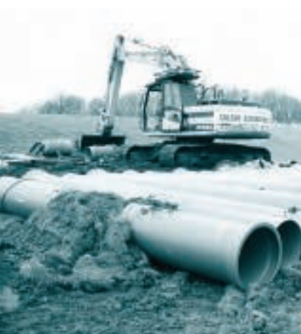
Water mains alterations at Shedfield Reservoir
