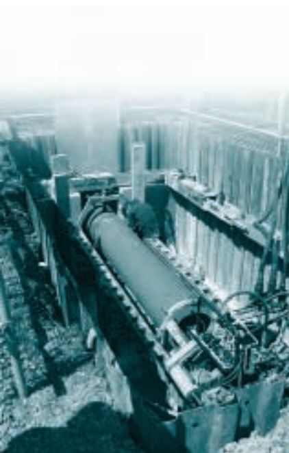
Pipe jacking a new water main under railway at Fareham
