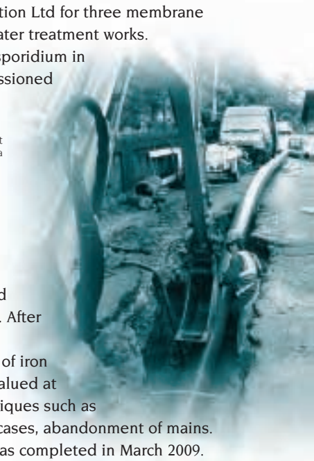
Slip lining a new water main at Highland Road, Southsea
