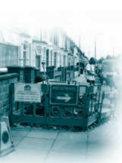
Repairing a water main
