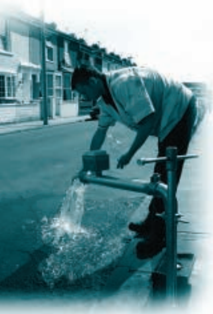
Checking water pressure flow
