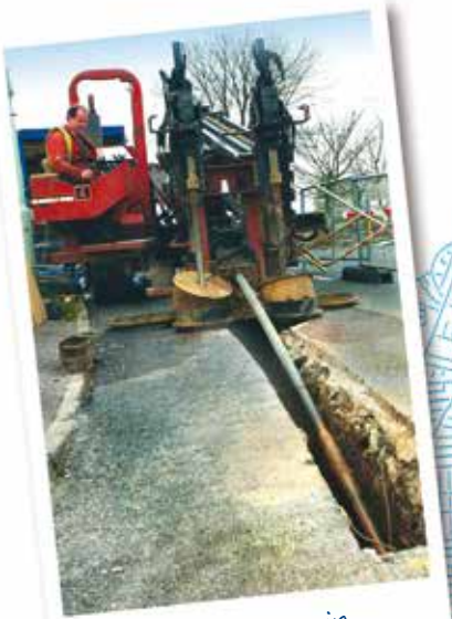
Laying a new main
