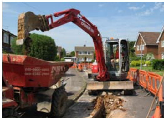
LEFT Mainlaying work being carried out by the Company's contractor
