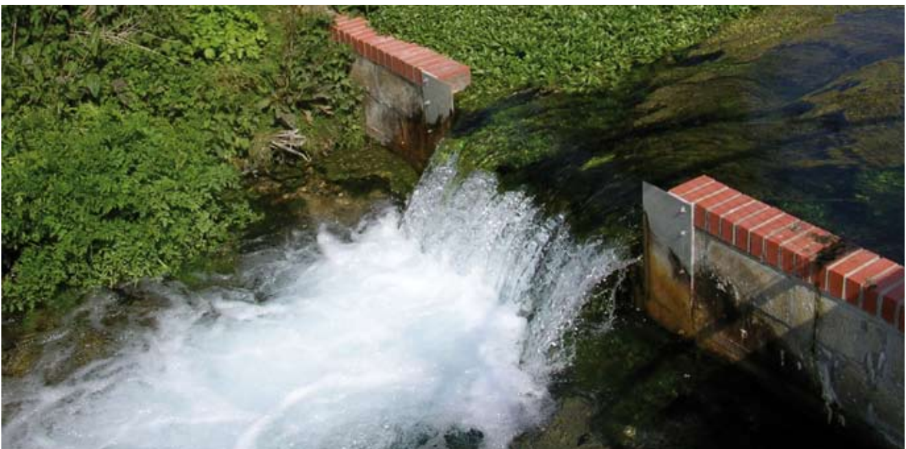
Flow of water over weir at Bedhampton Springs source
