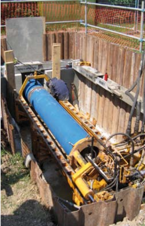
ABOVE Pipe jacking of water main under railway line embankment
