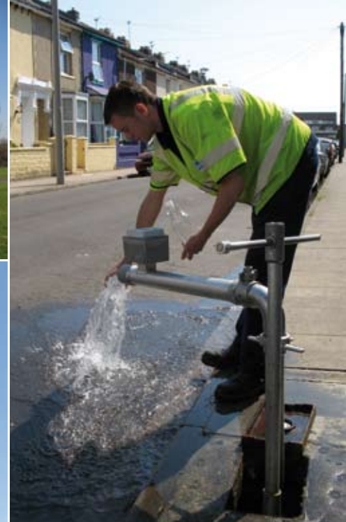
ABOVE Checking pressure of mains water
