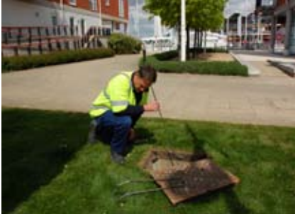
Leakage detection work at Gunwharf Quays, Portsmouth
