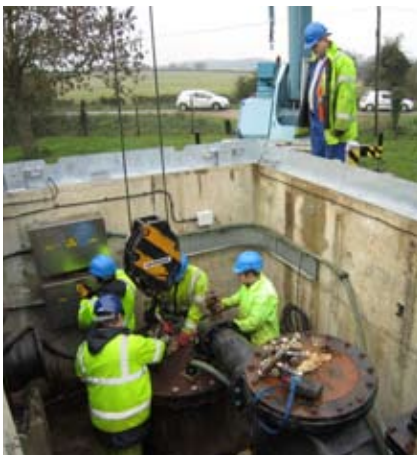
Changing a borehole pump at Lavant Water Treatment Works
