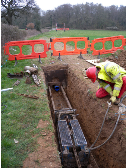
Pipe bursting of water mains being carried out as part of the Purbrook Heath mains renewal scheme
