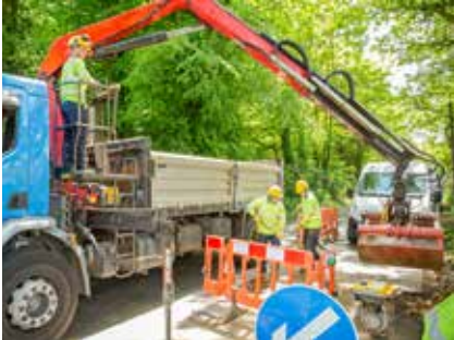
Portsmouth Water staff carrying out maintenance work on the mains network.
