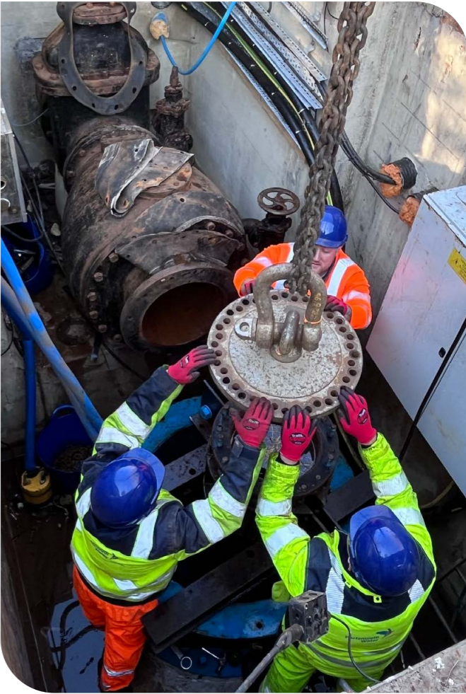
Northbrook pump replacement
