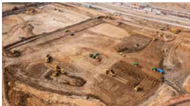
Figure 6. March 2025 marked the beginning of the 'big build' phase of the project, with construction underway for a 230m concrete culvert and the embankment ground improvement zone
