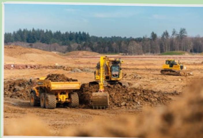
Havant Thicket Reservoir construction started in 2025
